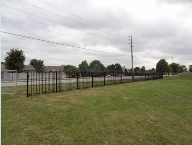
New Perimeter Fence Started
