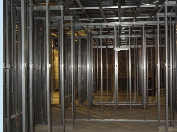
Army - 1st floor framing
