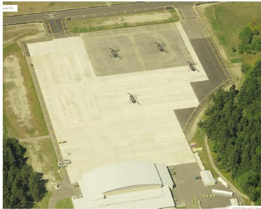
Ft Lewis, WA – Chinook Hangar and Apron
