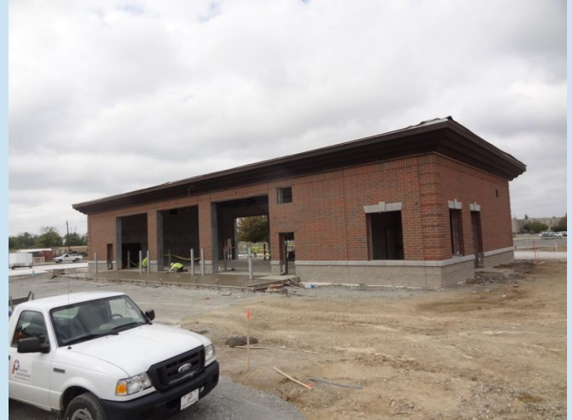
Entrance slab being placed
